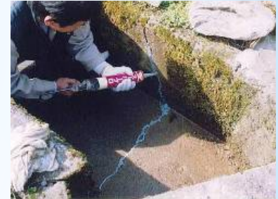
Repairing cracks on a dike
