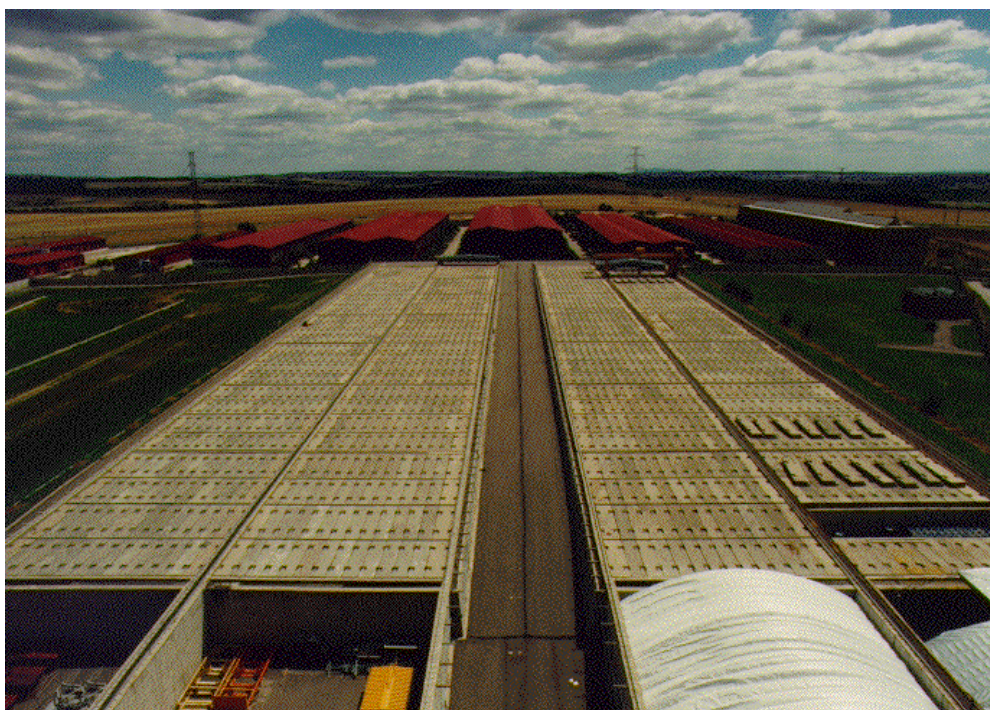
Figure A2.2 Dukovany LLW and ILW Repository
