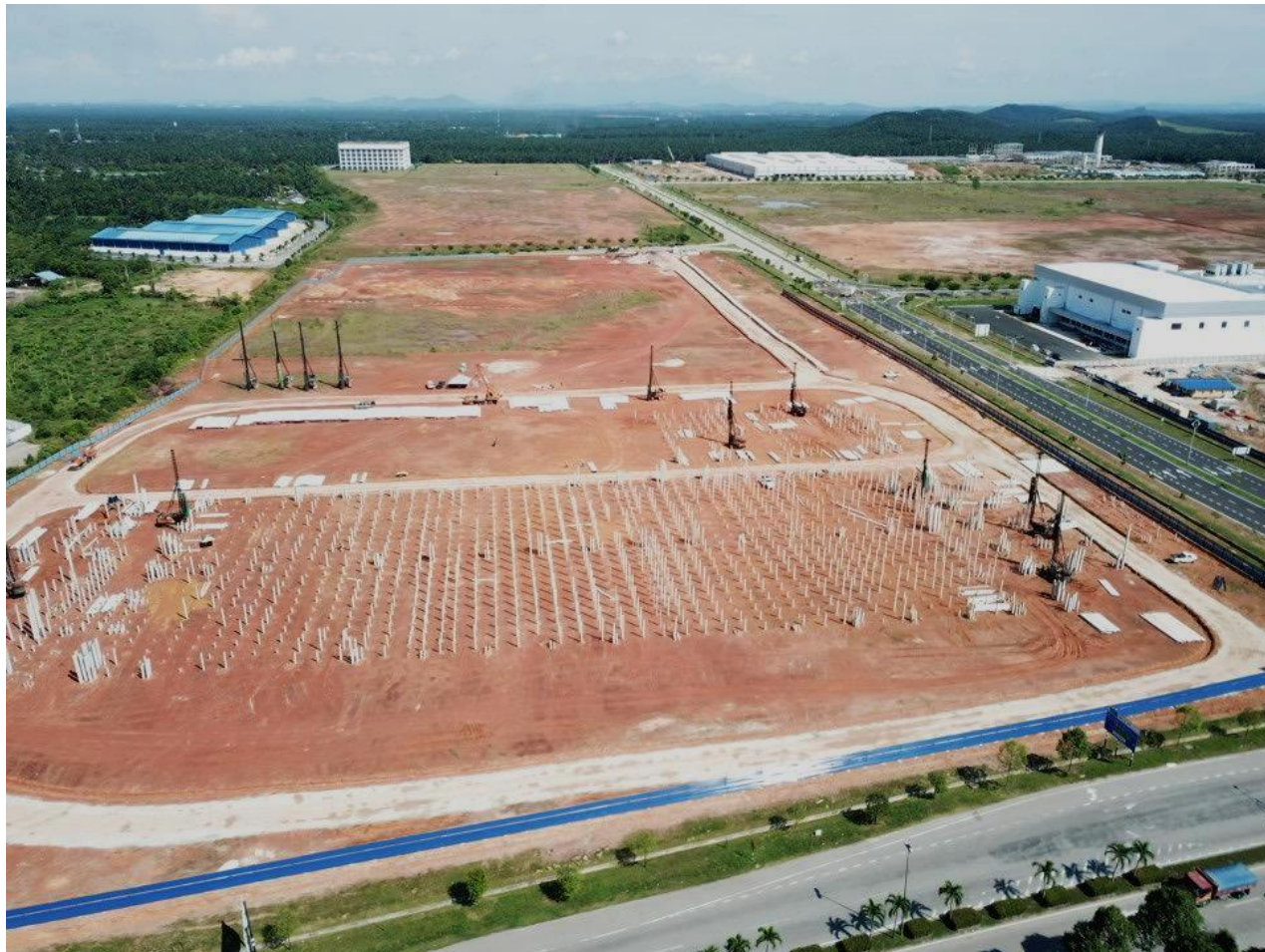
PILING WORKS | 08 October 2020
