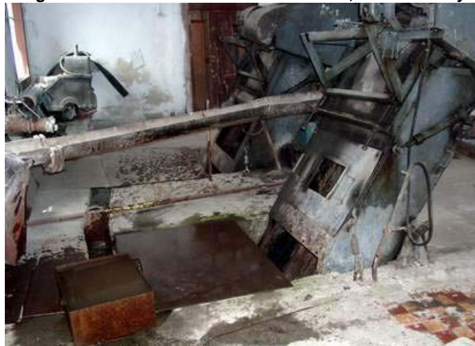
Figure 2.3 Screens with mechanical rakes, Vanadzor city
