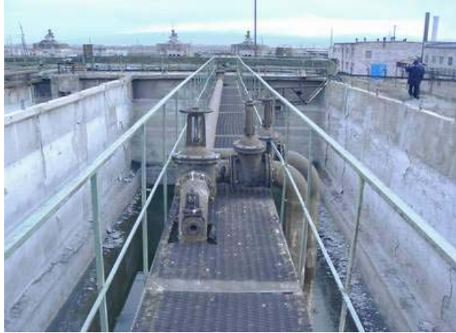
Figure 2.6 Aerotanks, Masis city
