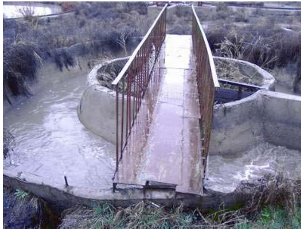
Figure 2.4 Tangential sand trap, Echmiadzin city
