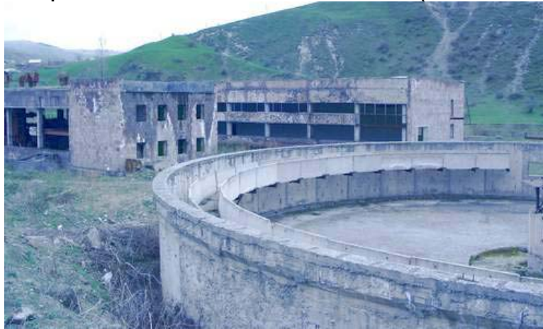
Figure 2.14 Uncompleted construction of the treatment facilities (the second stage), Vanadzor
