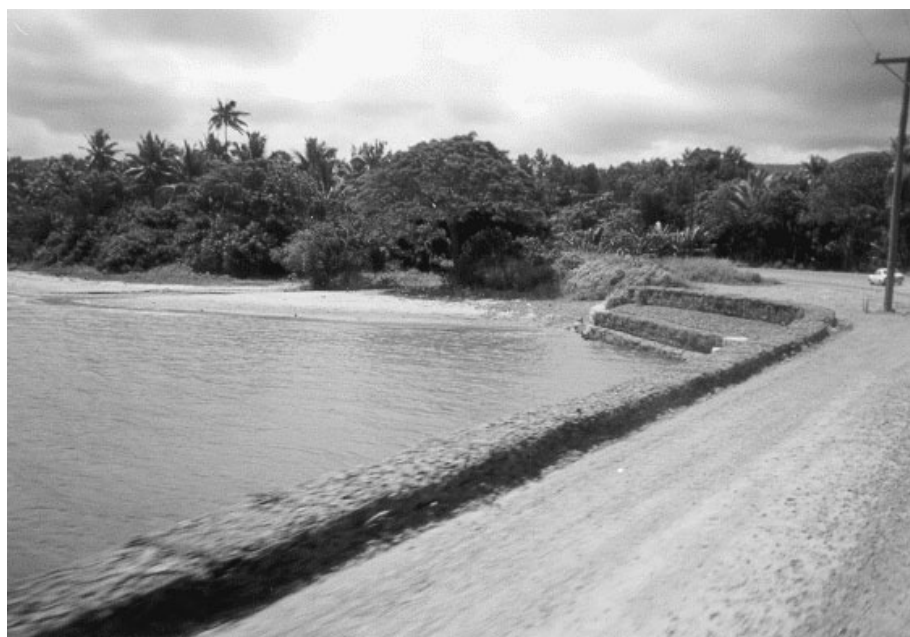
Figure 11. Seawall along the coral coast
