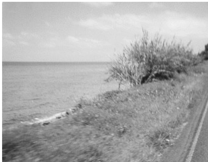
Figure 10. Stretch of road near Suva close to the high water mark
