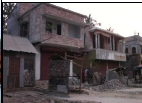
demolished and rebuilt shops
