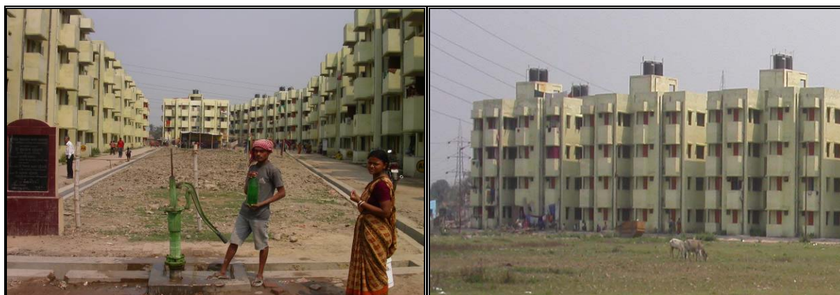
One of the Project's relocation sites: VAMBAY housing in Nonadanga, Kolkata
