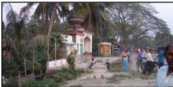
Demolished temple along the road (SH1)
