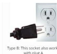
Type B: This socket also works with plug A
