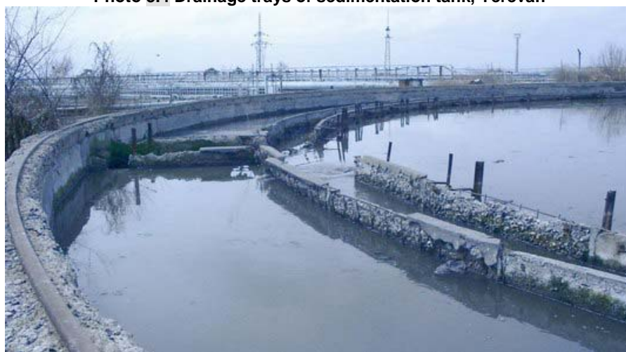
Photo 3.4 Drainage trays of sedimentation tank, Yerevan
