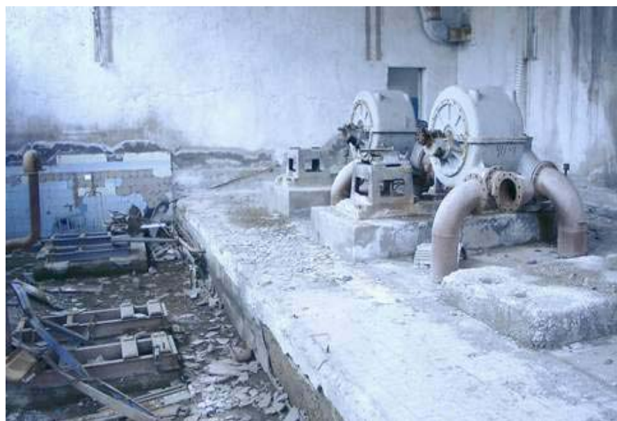
Photo 3.4 Drainage trays of sedimentation tank, Yerevan
