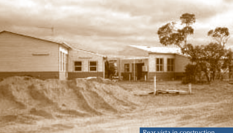
Rear vista in construction
