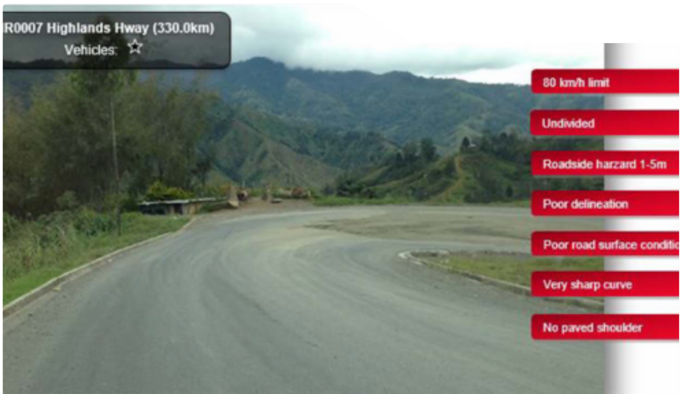
Example of a one star rated road for vehicle occupants; 91 per cent of the 571km corridor Highlands Highways was assessed as being in this category.
