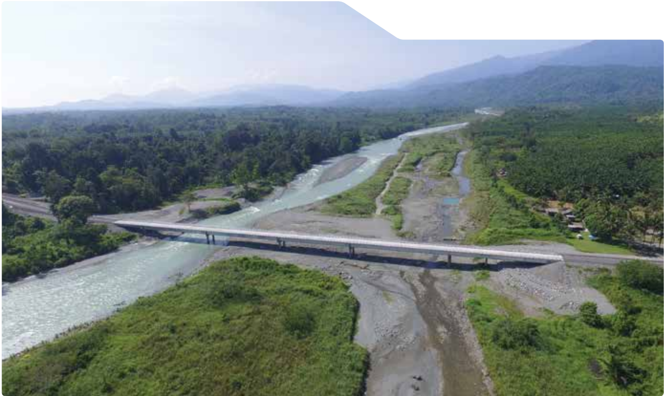
Kumusi Bridge, Oro Province. TSSP supported the design and construction of four bridges costing PGK82.2 million in Oro Province after Cyclone Guba destroyed most of the bridges and caused significant damage to other infrastructure in 2007. At 285 metres in length, the Kumusi bridge is Papua New Guinea's longest two lane bridge.
