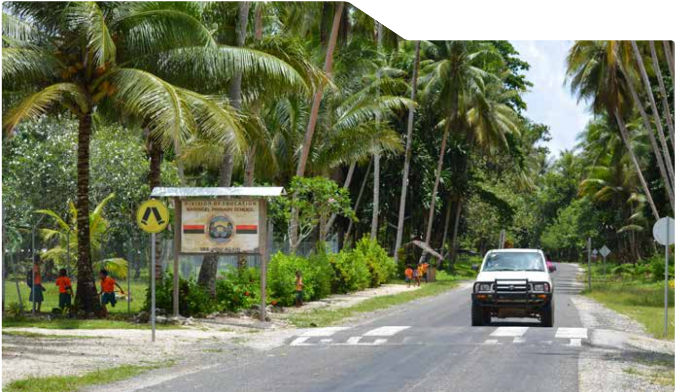
An example of the discrete road safety features TSSP has introduced in its upgrade of the Momote to Lorengau Road on Manus Island.
