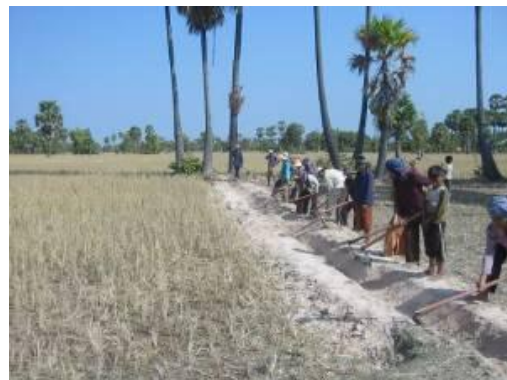
Construction of a quaternary canal by a local farmers' group
