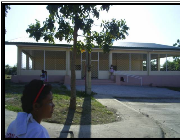
A community center in KV III, Trece Martirez City
