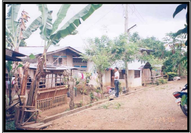
Streets in the Nazareth site were lined with open drainage lined with concrete hollow blocks, not underground like in the Mulanay site.
