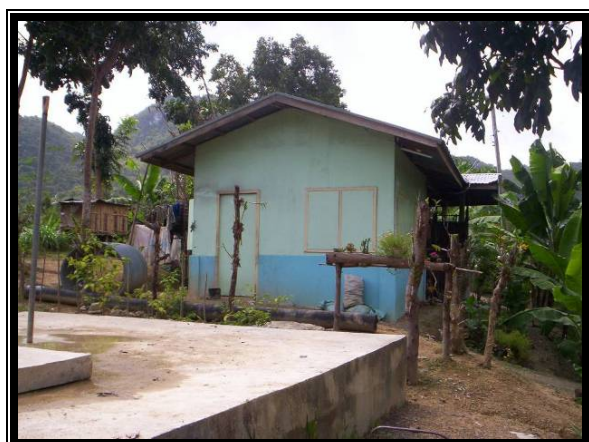
Core house (4m x 4m) in the resettlement area
