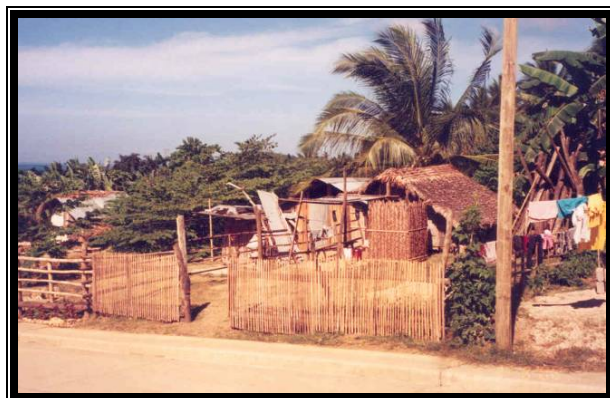
Resettlers in Mulanay utilize local organic materials in the absence of financial assistance in house construction.
