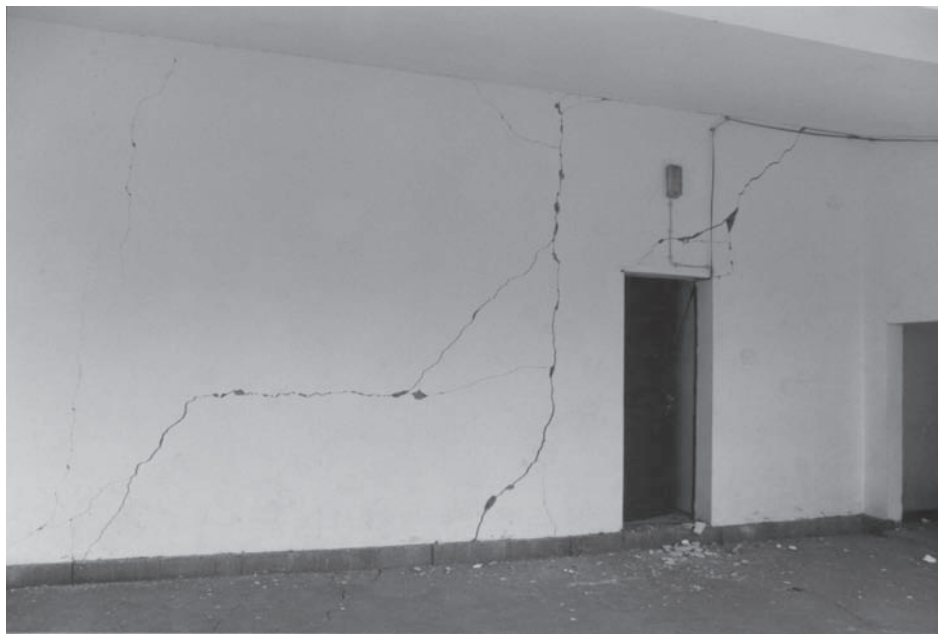
Figure 8.4. Damage in reinforced-concrete roof beams and in retaining walls at school in Ribeirinha
