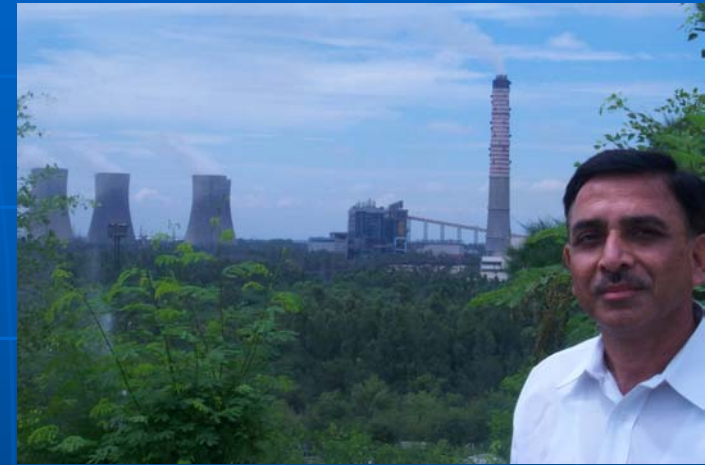
Heat rate efficiency in power plants improved under the Greenhouse Gas Pollution Prevention Project in India. (John Smith-Sreen, USAID/India)
