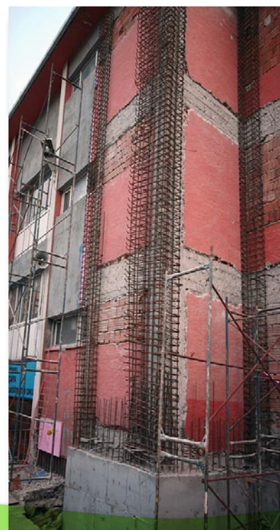
A school building in Istanbul being retrofitted by ISMEP
